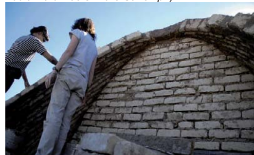
Figura 15. Bóveda nubia, taller de construcción. (Fuente: The Swan House and Adobe Construction Lab Sales Presentation . Presidio, Texas. Big Bend Country, reachable by scenic route only. Workshop Photos. Workshop Photo Archive 2005 - 2008).
