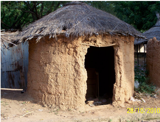
Figure 2. Southern Nigerian Compressed Earth Block Building. 7
