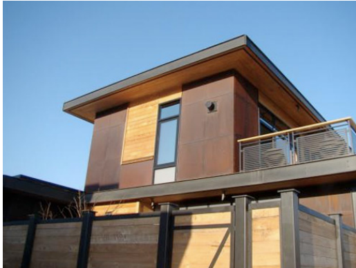
Figure 4. Rammed Earth Wall Building. 9
